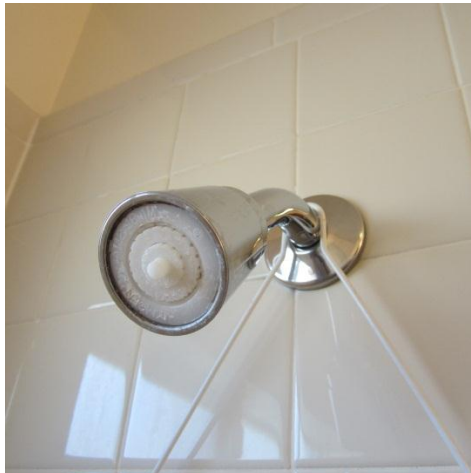
Typical 2.5 GPM Showerhead Used in Apartments
