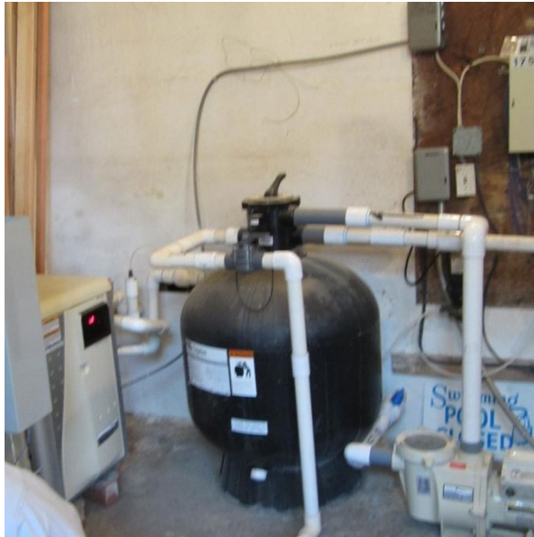
Pool Heater and VFD Pump for 175 Albion
