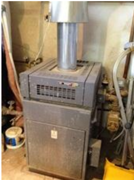
250KBTU Boiler 2 of 2 for 195 Albion
