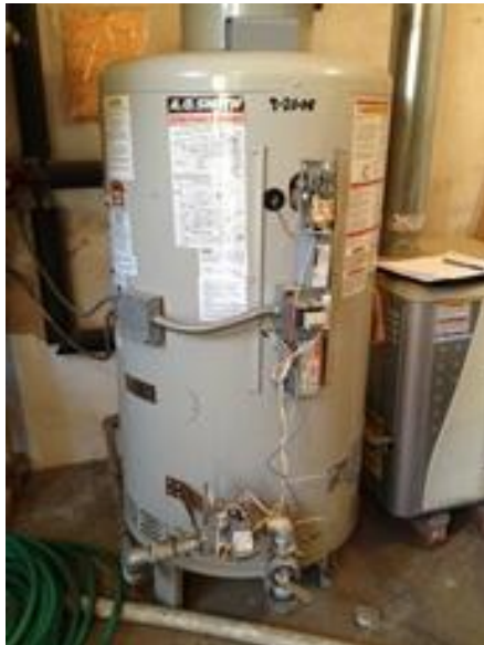
660KBTU Boiler 1 of 2 for 195 Albion
