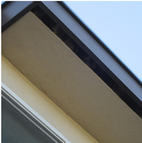
Uninsulated Flat Roof Cavity with Perimeter Soffit Venting
