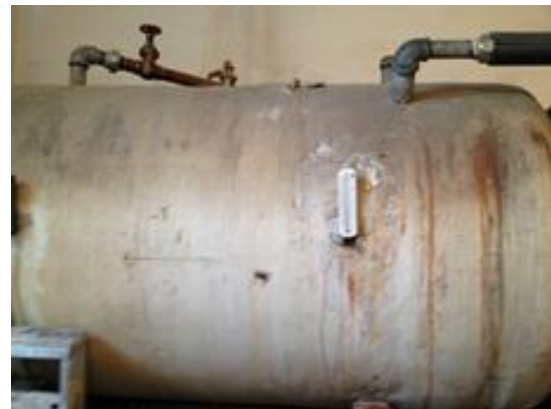
Figure14: Storage Tank for Boiler 1 of 2
