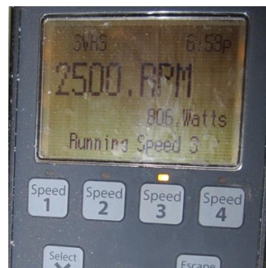
175 Albion Pool Pump VFD Display
