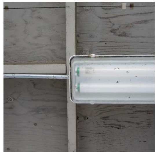
T12 Linear Fixtures in Carport
