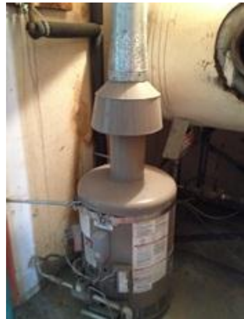
200KBTU Boiler and Storage for 175 Albion
