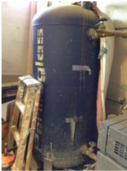
Uninsulated Storage Tank for Boiler 2 of 2 for 195 Albion
