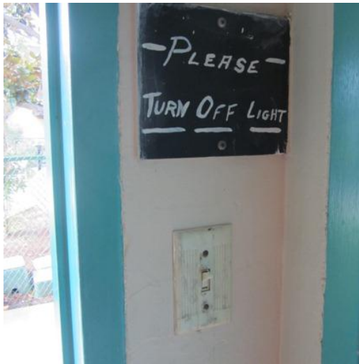
Common Area Hall Lights are Manually Switched
