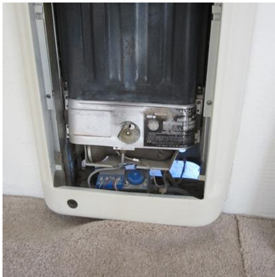
Original Natural Draft Wall Furnace in Apartment
