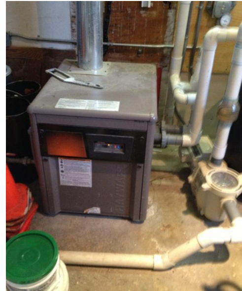
Pool Heater and VFD Pump for 195 Albion
