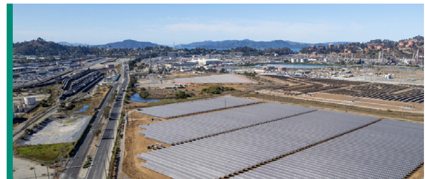
MCE's 10.5 megawatt Solar One in Richmond, California powers almost 4,000 homes annually and supported over 300 jobs
