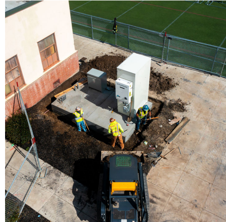
Battery installation at Pittsburg High School
