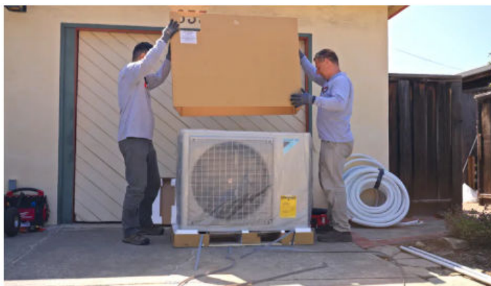
Contractors get ready to install an electric heat pump at a home in the San Francisco Bay Area. (Silicon Valley Clean Energy)
